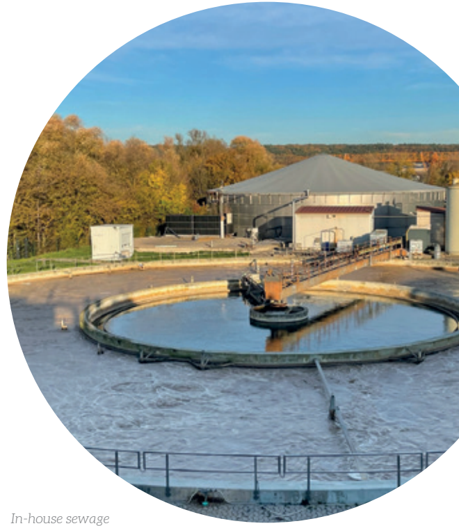
In-house sewage plant in Zapfendorf
